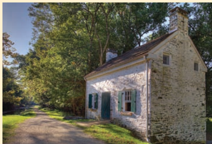
Exterior view of Lockhouse 22. Courtesy Chris Hanessian, C&O Canal.
